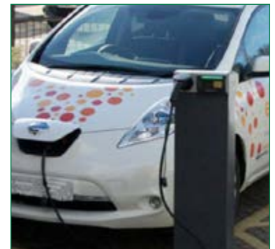
Installing electric vehicle charging
