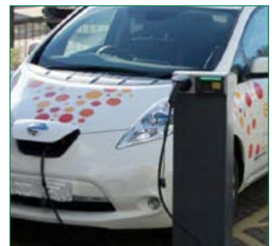
Installing electric vehicle charging
