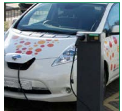
Installing electric vehicle charging
